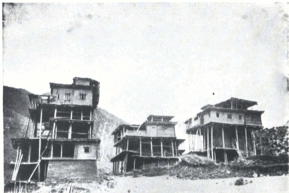
TIBETAN HOUSES OF YELLOW MUD, BUILT VERY MUCH LIKE MEXICAN ADOBE HOUSES
